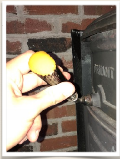
Open main damper
